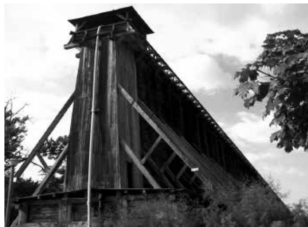
Fig. 2. Cooling Tower in Czechochynek (Poland)
